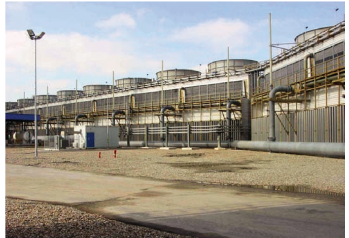
Wet-Dry Hybrid Cooling —The wet-dry hybrid cooling tower offers efficient cold water temperatures with reduced visible plume and enhanced water conservation.
